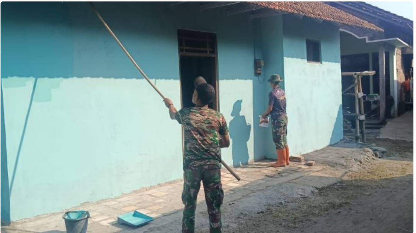
(Foto istimewa) Pengecatan RTLH TMMD 116 Kodim 0722/Kudus
